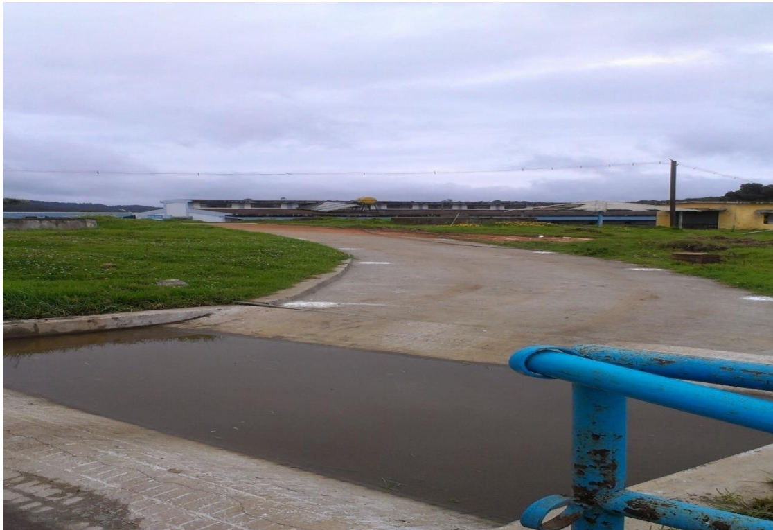
Tyre Dip at Entry
